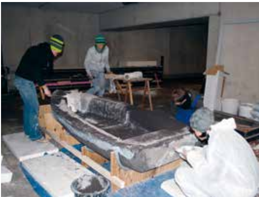
Concrete lamination process
