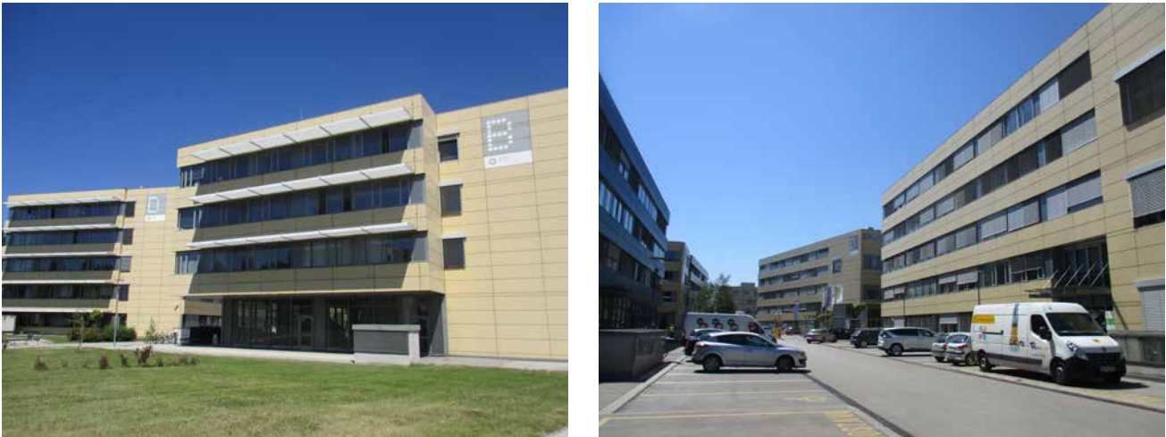
FIG. 3.2 Comprehensively designed urban and architectural concept as a consequence of an efficient professional approach and quality design conditions (Technology Park Ljubljana).
