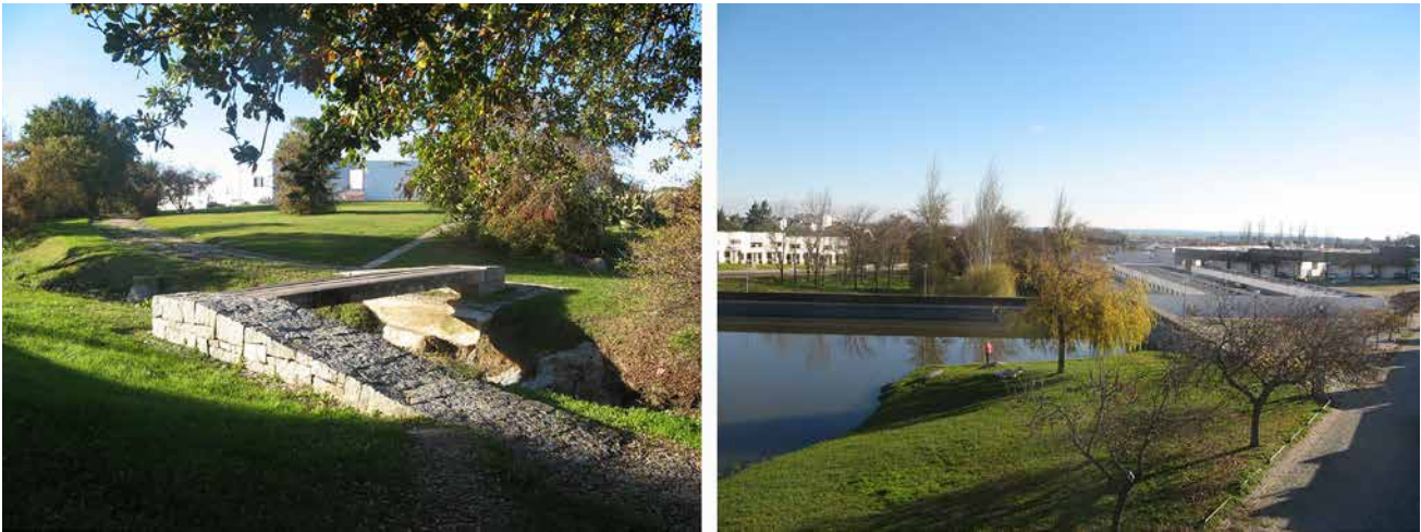
FIG. 3.3 Quinta da Malagueira by Álvaro Siza, Évora, Portugal ( Images by author, December 2011 )
