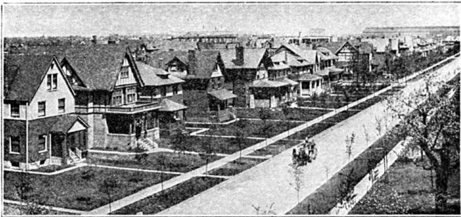
THE BUILDING OF GARY.
