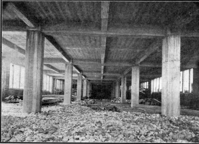
MESSRS. D. JONES' NEW FACTORY, SURRY HILLS.
