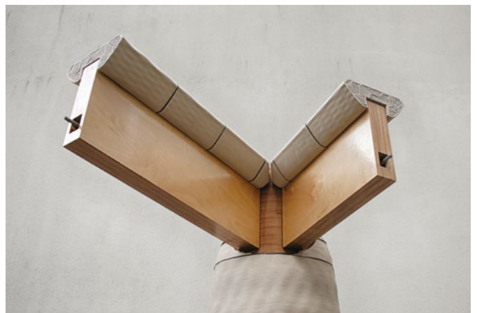
Figure 7: Connection between beams and columns.
