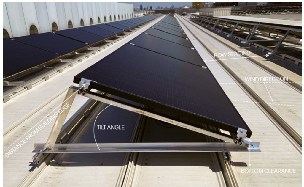
Figure 2: Typical geometric parameters for flat-roof mounted PV strings.
