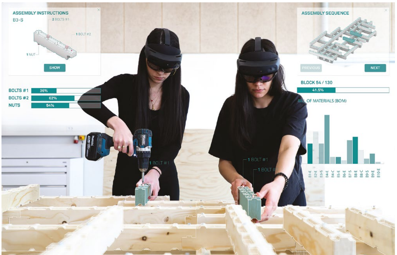
Figure 6: Cyber-physical collaborative assembly of ReconWood structures aided by Mixed Reality.
