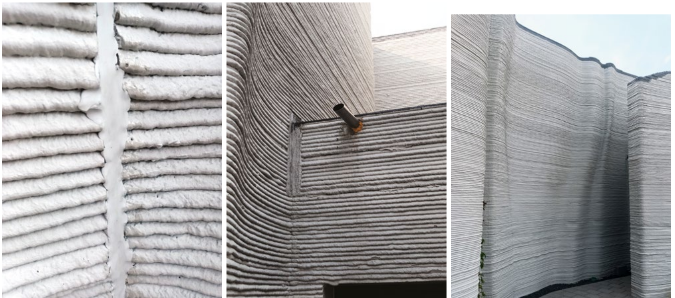
Figure 4: Images of a 3D-printed building in Heidelberg, Germany. From left to right: spout in construction foam, expansion joint in 3D printed wall, parapet finish with liquid plastic sealant.
