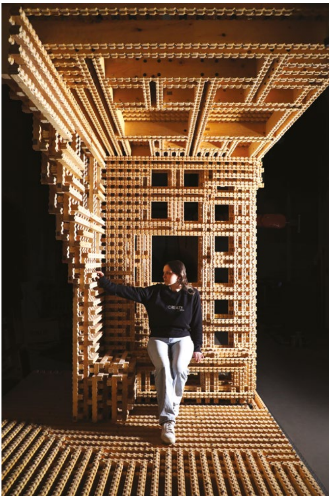
Figure 7: ReconWood architectural demonstrator showcasing the integration of wall and slab structures.
