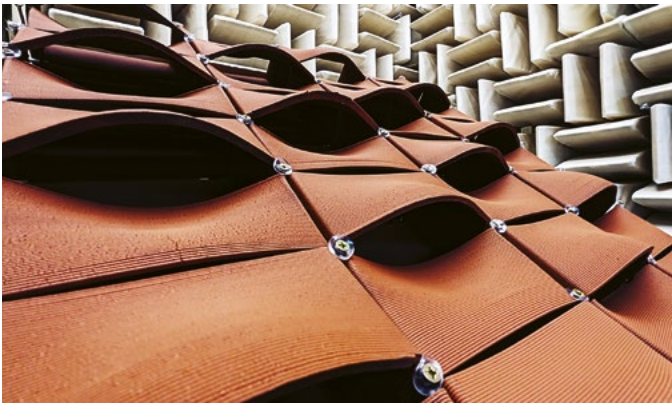
Figure 5: Additively manufactured acoustically effective ceramic facade [85].
