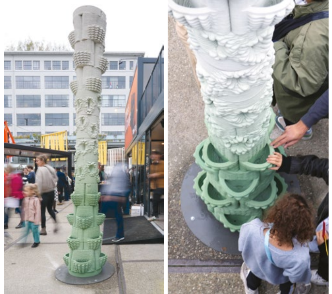
Figures 10-11: Assembled 3D concrete printed column showcased at Dutch Design Week 2024.
