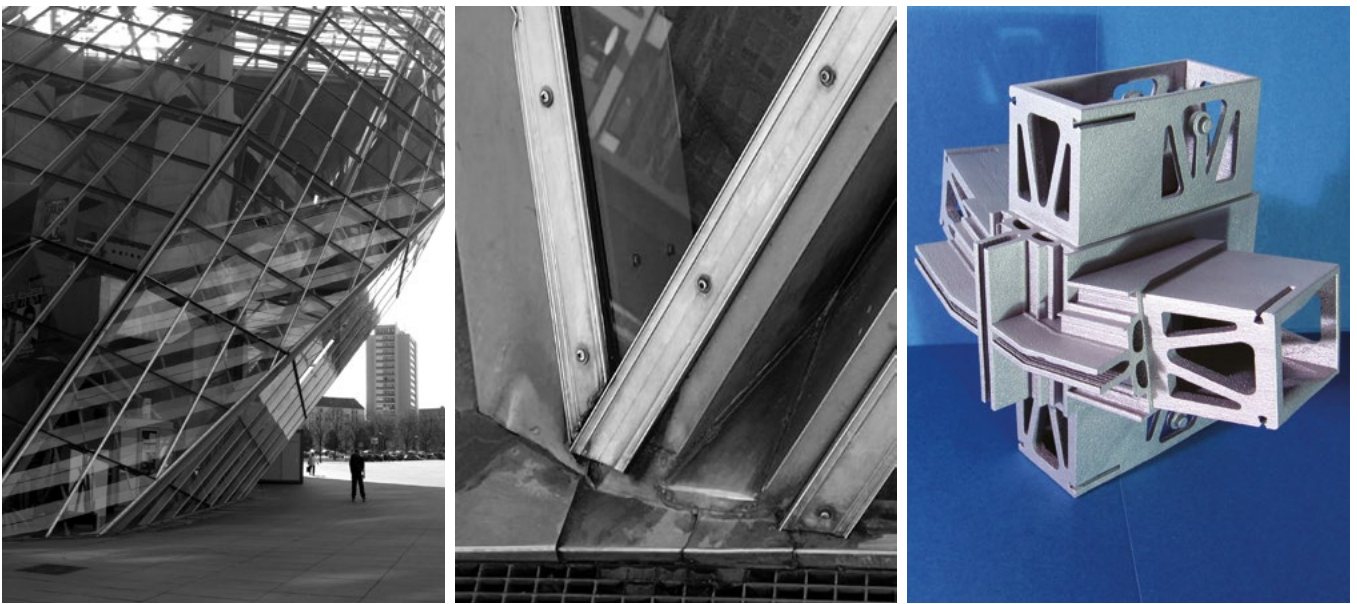
Figure 1: from left to right: challenging geometry, problem detail (unsolved), prototype of the AM solution "Nematox II" AM-Façade node (H. Strauß, 2010).
