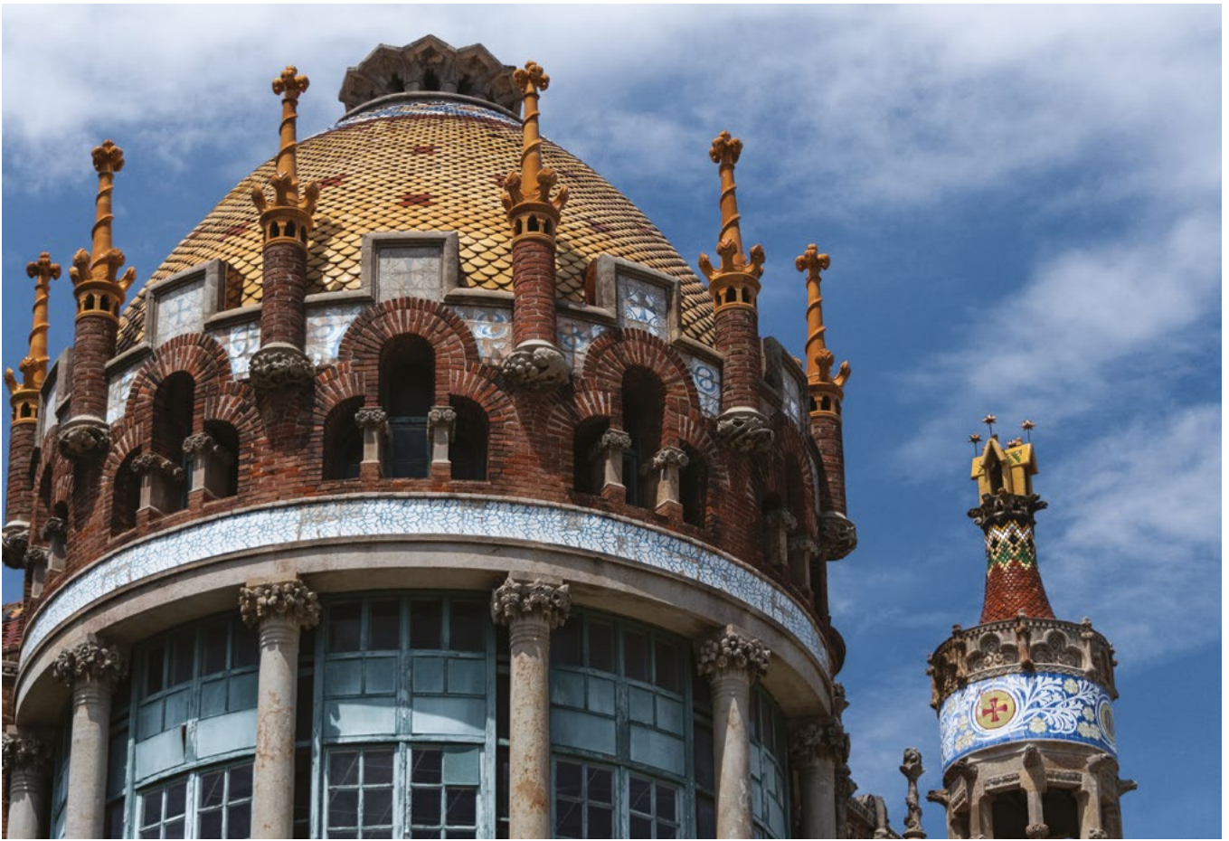
Figure 1: The versatile use of ceramic components in a facade. Klinker Bricks alongside glazed tiles and roof tiles, as well as ornaments such as pinnacles. (Hospital de la Santa Creu i Sant Pau, Barcelona, Spain).
