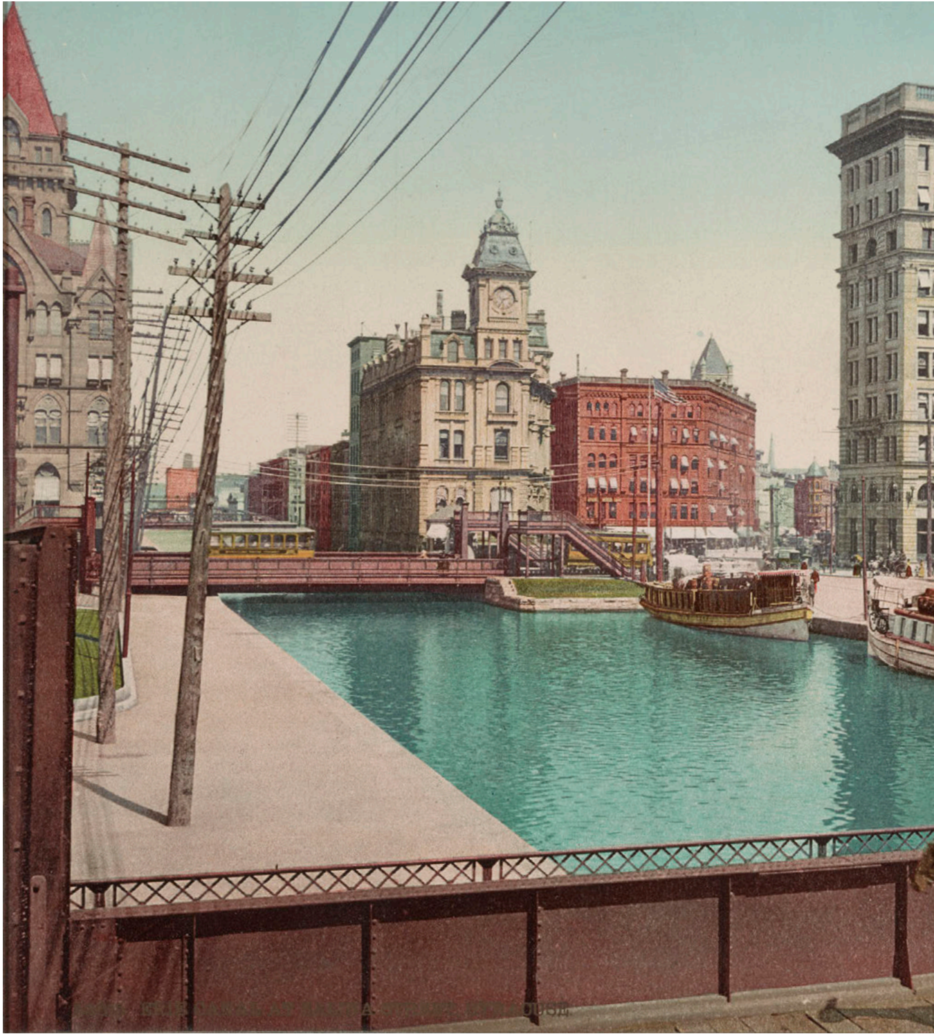
^ Fig. 3 Erie Canal at Salina Street, Syracuse, Detroit Publishing Company, c. 1900 (Source: Courtesy of the Library of Congress, no known restrictions on publication)
