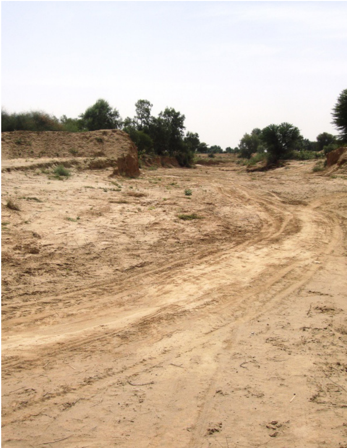
^ Fig. 3 Earthen diversion structure at Bhaati Spate River, DG Khan, Pakistan. The site is more than 250 years old (Source: Karim Nawaz, 2006).
