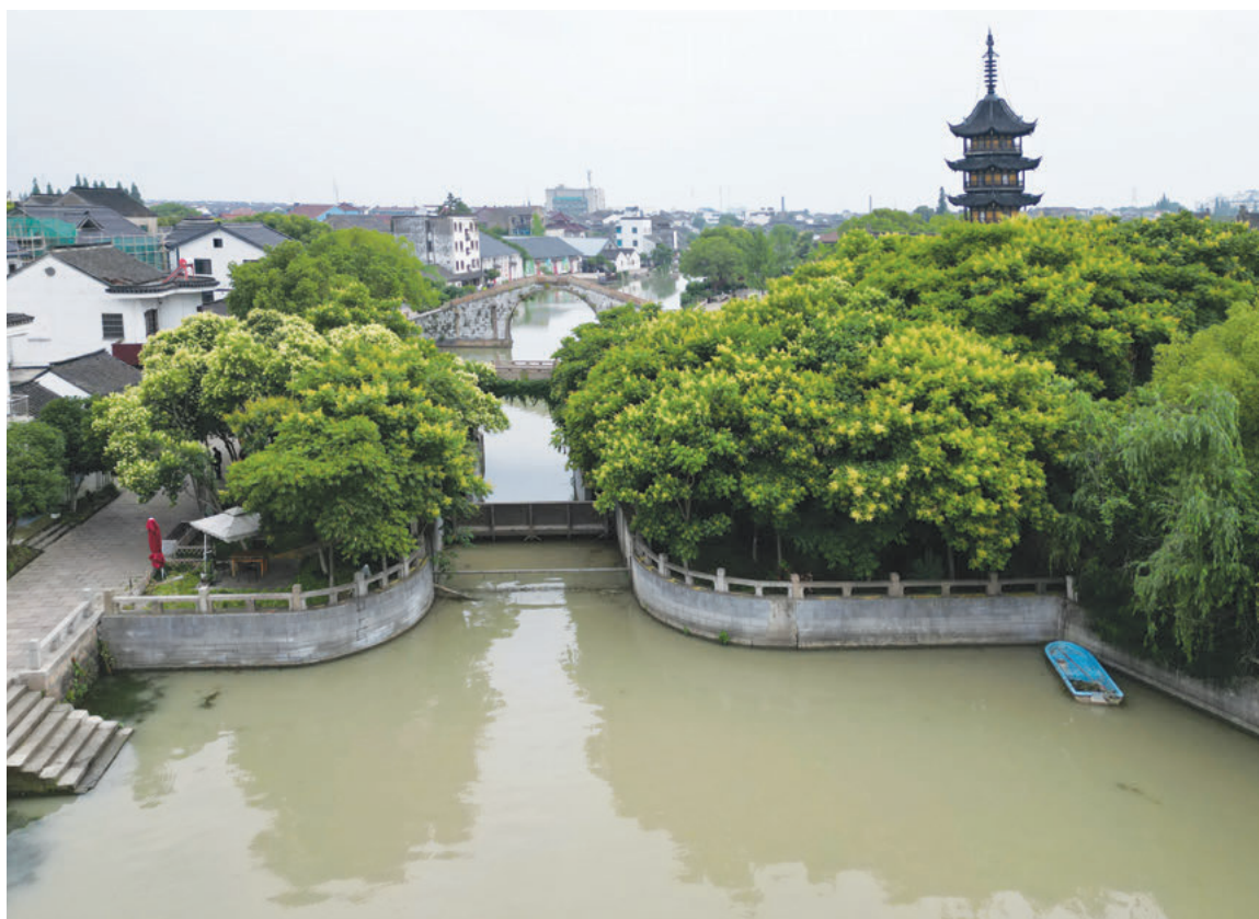
^ Fig. 6 The addition of modern sluices between the polders forms weiqu . The entrance of Zhenze is now demarcated by a sluice (added in 1997) near the ancient Yuji Bridge (Source: Wei Lei, 2023).
