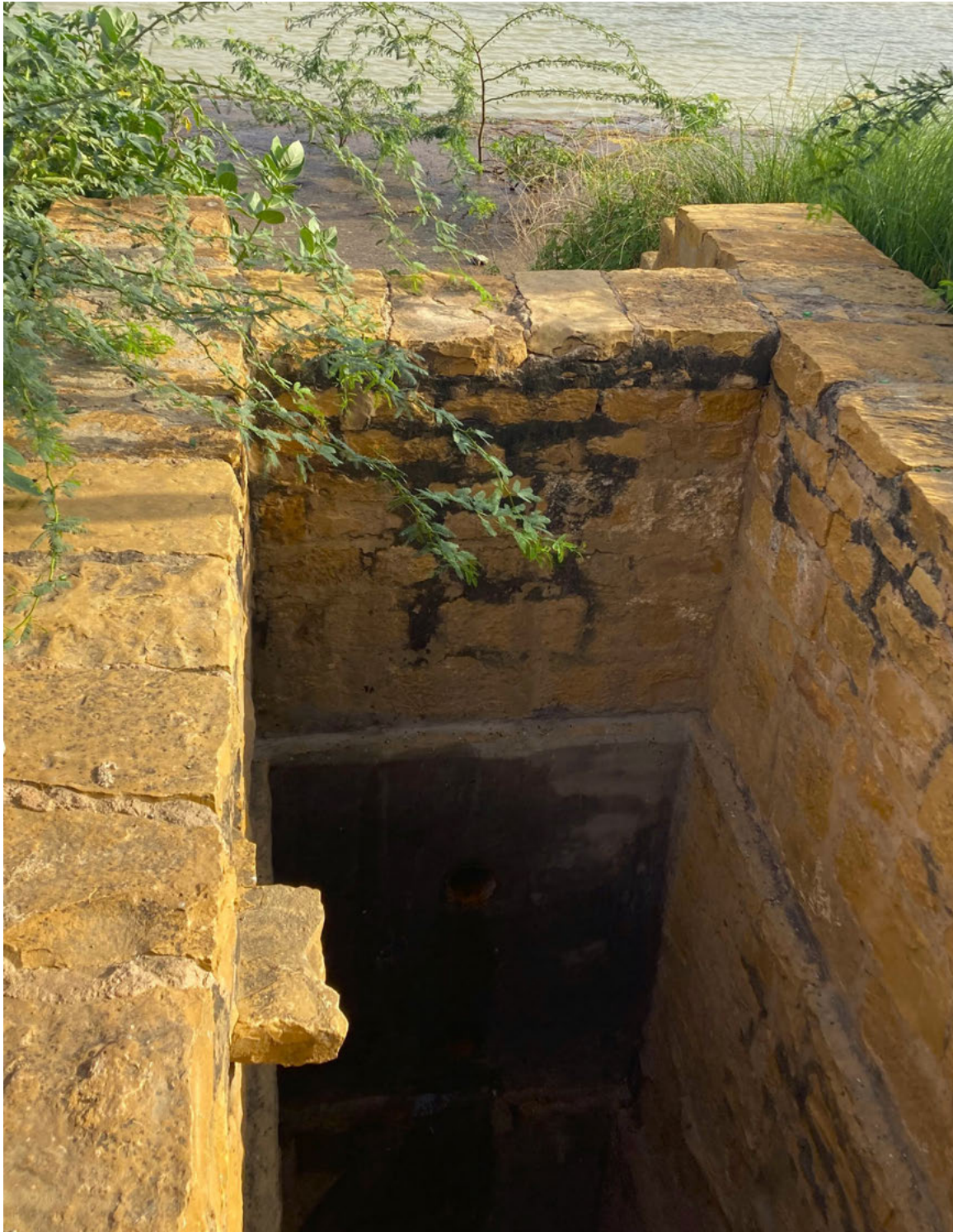
^ Fig. 6 Outlet shaft at the Bada Bagh Khadeen (Source: Pierantonio La Vena, 2023).
