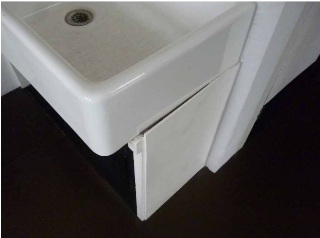
FIG. 5.2 Deformation of thin timber elements of furniture
