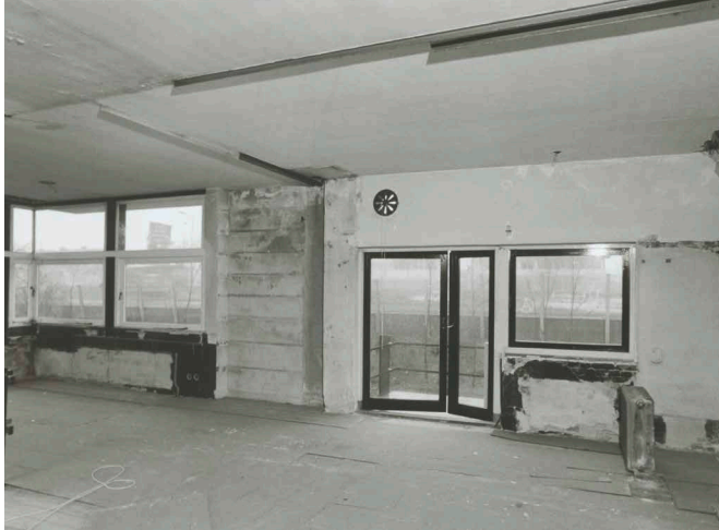
FIG. 3.3 The partially dismantled upper floor
