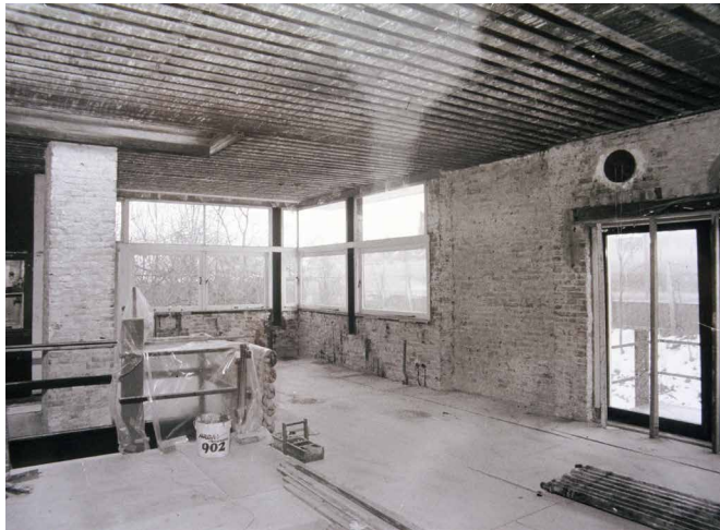
FIG. 3.5 The upper floor of the Rietveld Schröder House in dismantled state
