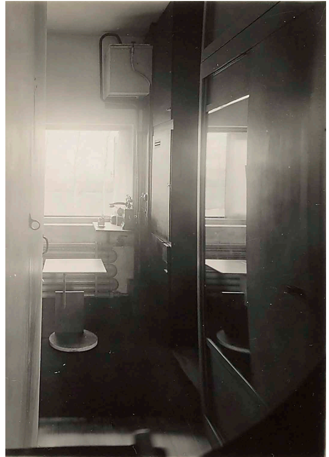
FIG. 4.8 Upper floor interior, Schröder's bedroom, c.1925
