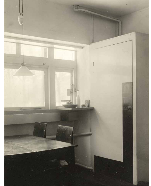
FIG. 4.43 Ground floor, kitchen with deliveries shelf, c. 1925
