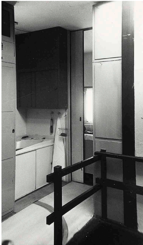
FIG. 4.23 Upper floor interior, bathroom with bathtub, c. 1925
