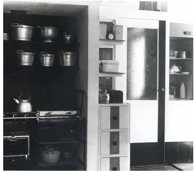
FIG. 4.46 Ground floor, kitchen, c. 1925
