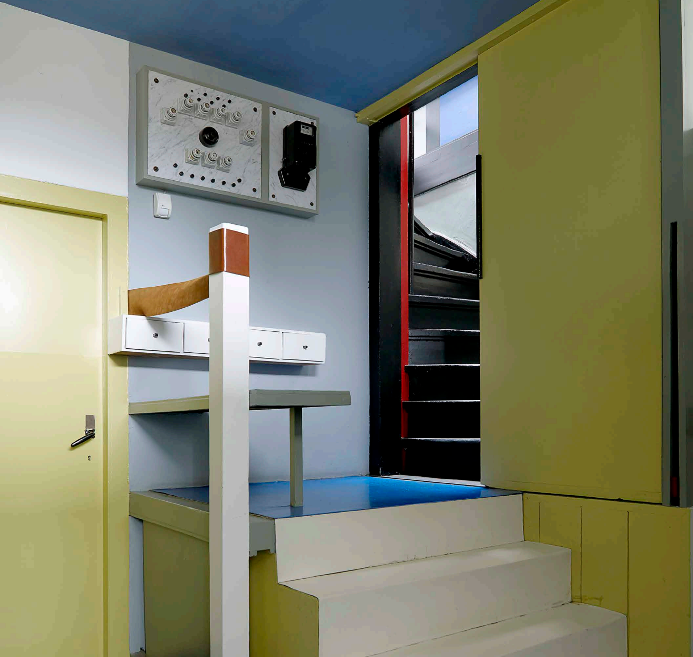
FIG. 4.30 Ground floor, hall with fuse box and platform, 2010
