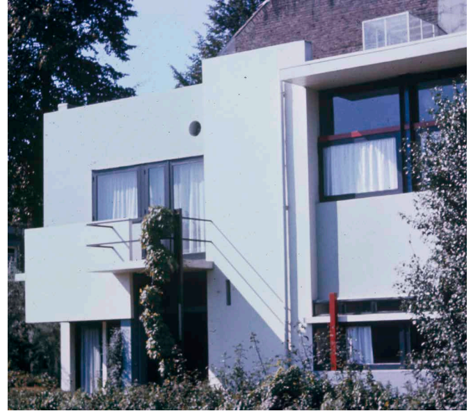
FIG. 2.5 A colour photograph from before the restoration shows that the greys had become bluish
