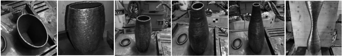
Figure 11: Manufacturing process of one column element.
