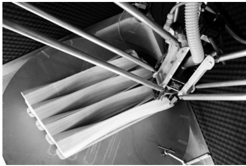
Figure 5: 3D printing process of one façade element (©Material Balance Research).
