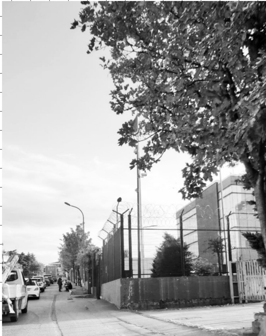
A well protected data centre in one of Istanbul's industrial regions, where taking photographs is not allowed even for the employees. Image by author.
