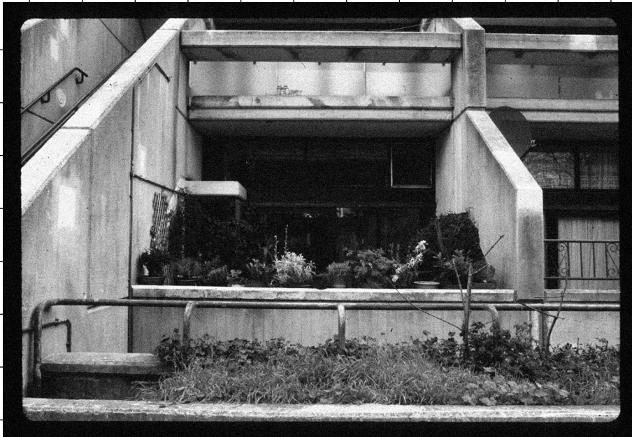
Alexandra Road. Photograph: Luis Diaz
