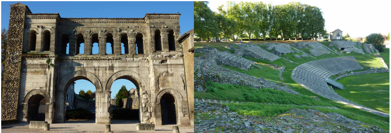
FIG. 4.7 The gate (left) and theater (right) at Augustodunum (Autun). The Saint-André gate is one of four Roman entrances into the city, situated at the cardinal points. Two remain complete and are still in use (image in the public domain, https://commons.wikimedia.org/wiki/File:Autun_porte_Saint-Andr%C3%A9.JPG ). The Roman theater was built in the first century CE during the reign of Augustus. It is the largest in France, with seating for 1500 spectators. Just outside the city walls exists another theatre, of similar size and age (image in the public domain, https://commons.wikimedia.org/wiki/File:Th%C3%A9%C3%A2tre_roman_Autun.JPG ).
