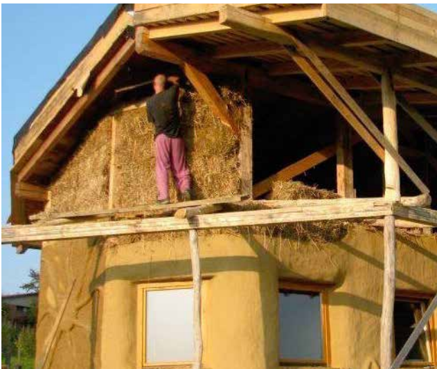
FIG. 4.2 A+B: Clay mortar plastering (images by Kristijan Zver, 2007)
