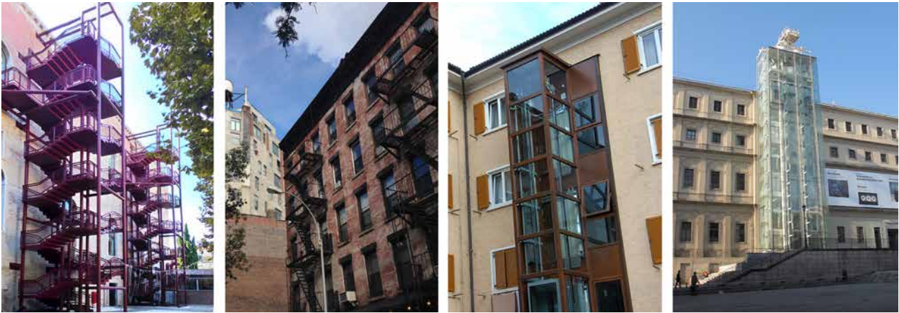
FIG. 3.2 Examples of functional additions for accessibility and security: architectural prosthesis. From left: security stairwell in a historical building, Tolentini, Venice; external security stairs in New York (Image by Lidia Savioli, 2015); external lift in Bolzano (Image by Comune di Bolzano, 2014); external lift in the Reina Sofia Museum, Madrid (Image by Valeria Tatano, 2014)
